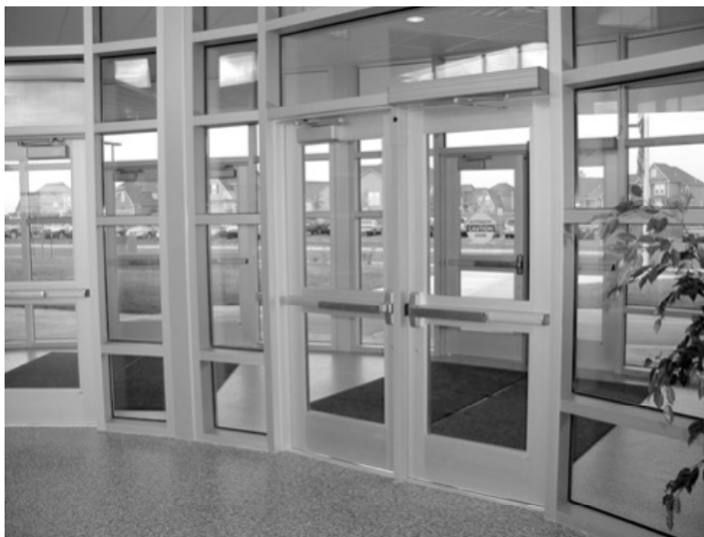
Main entrance at Ravenwood School allows exiting through multiple doors equipped with Von Duprin exit devices. LCN power operator on door at right accommodates those with disabilities.
