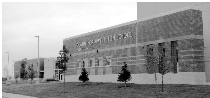
Olathe Northwest High School is one of four high schools in the Olathe district that all have the keyless entry system.
