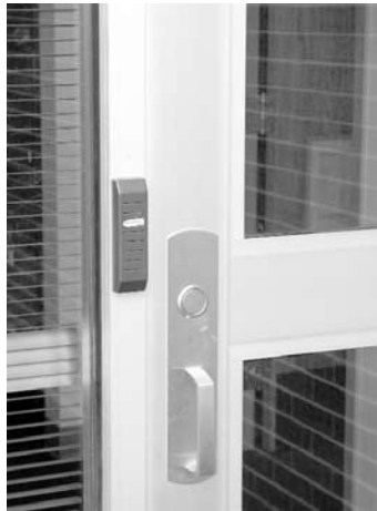
Dummy cylinder in outside trim restricts re-entry from playground to teachers and staff members with card credentials.
