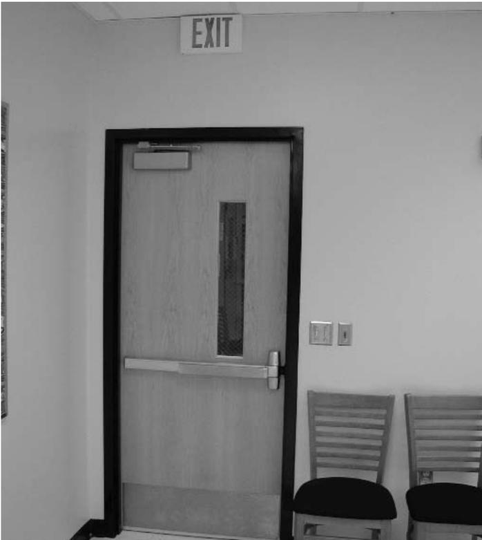
Von Duprin 99 Series exit device provides a safe emergency egress path on this interior door, while LCN door closer maintains security by keeping the door closed properly so it latches.
